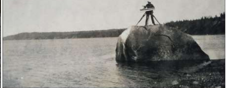
Figure 5. Coast Survey plane table mapping. The surveyor is using the plane table on an offshore rock in Cook Inlet, Alaska, circa 1910. The alidade can be seen on top of the surface of the plane table (U.S. Coast and Geodetic Survey c. 1910).
